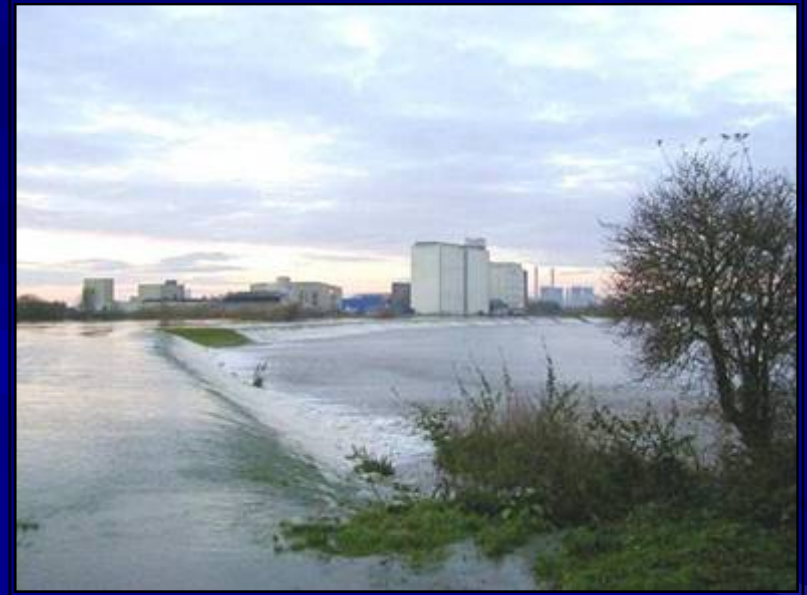
River Trent Overtopping Flood Banks at Beckingham Marshes, Gainsborough (photo Environment Agency)
