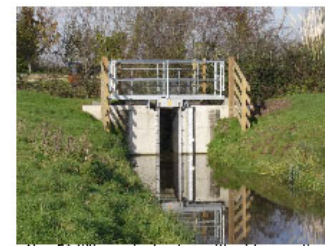
New EA tilting weir structure with wide operating range - Southlake Sluice
